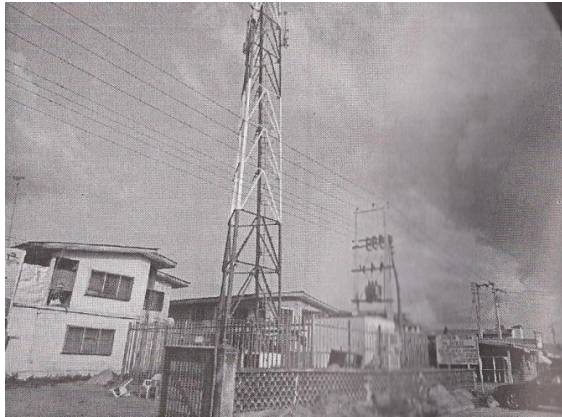
Figure 2. A telecommunications tower in front of residential buildings. Adelusola (2013:20).
